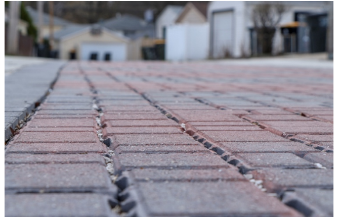
The green alleys in Wauwatosa feature permeable brick pavers. Installed with gravel in between the pavers, water can flow between the pavers, through the gravel, and infiltrate back into the soil. Photo credit: City of Wauwatosa
