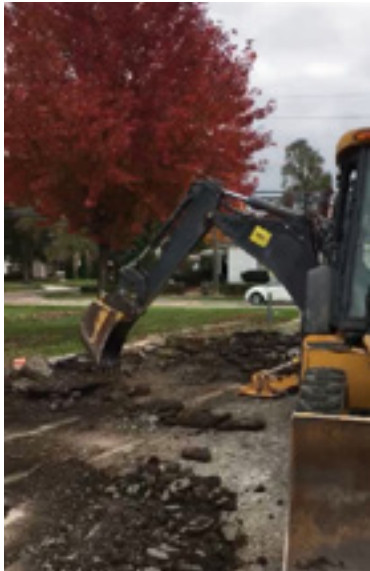
Contractor removal of asphalt
