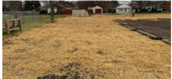
Seed and straw laid after depaving.
