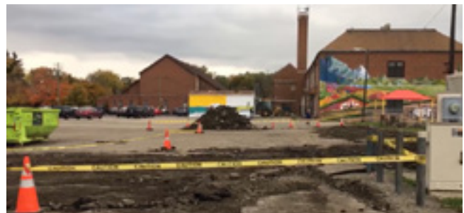
Removing asphalt and debris.
