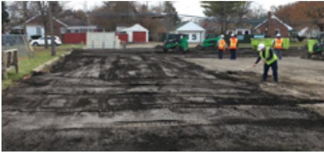
Backfilling topsoil into the depaved area.
