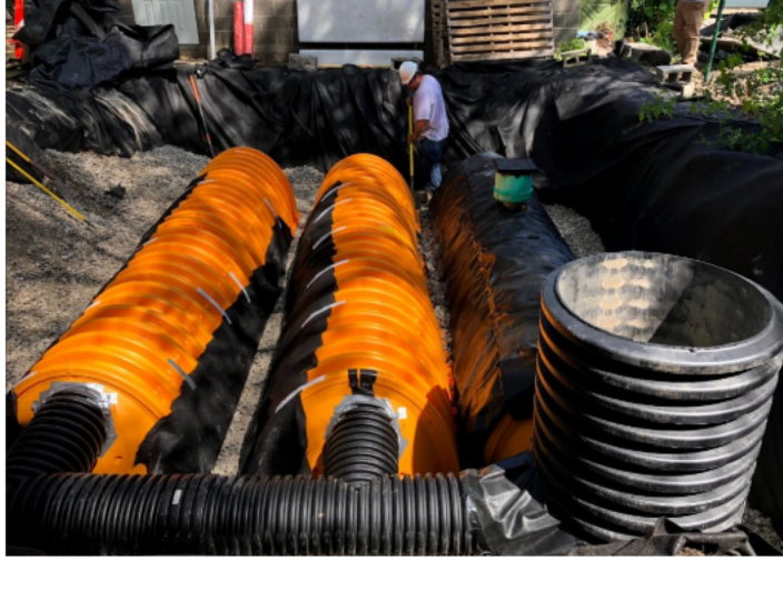
PizzaPlex , a "community pizzeria" located in Southwest Detroit, implemented a modified Stormwater Cistern lot design, building an underground system that allows rainwater to be infiltrated into the ground, staying out of our sewer system. This helps keep the Detroit River clean during large storm events!
