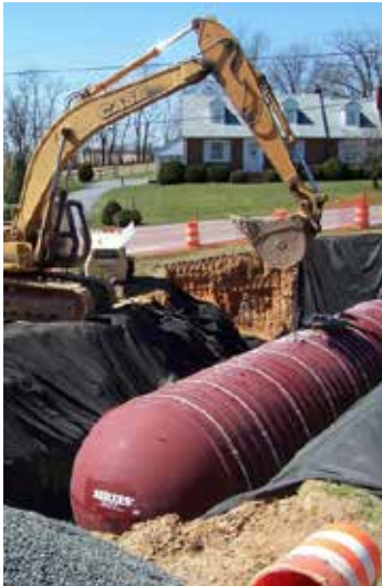
1 - Installation of below-ground cistern
